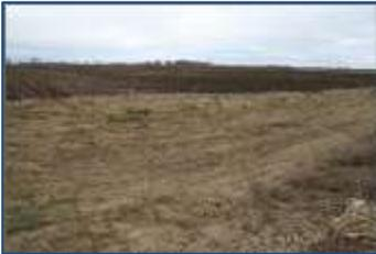
This basin, located above Lake Augusta near Norton Ave on 100th Street NW (Wright County), serves to slow the flow of water downhill to Lake Augusta. This basin was constructed to correct a developing erosion problem that was sending a large amount of sediment into Lake Augusta. By allowing runoff to pond in the basin during rain events rather than gouging the hillside, sediment is kept on the land instead of in the lake.
